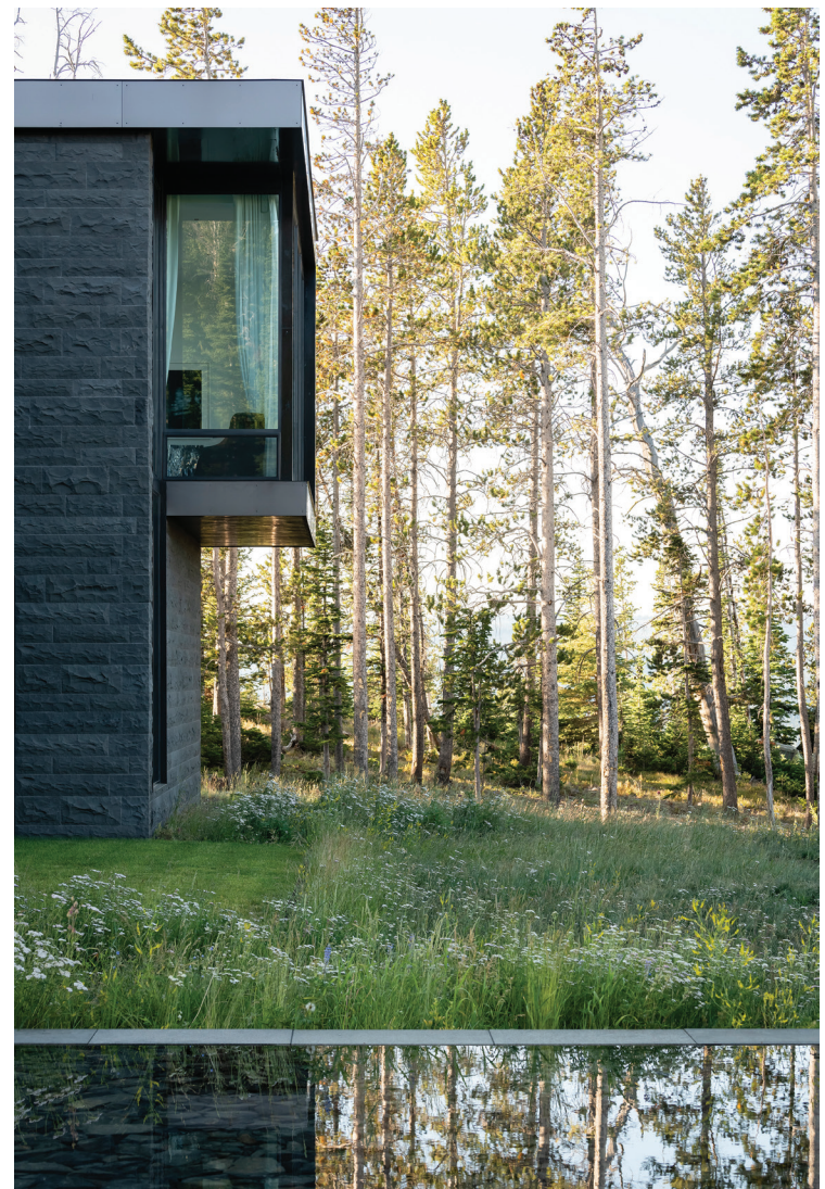
THIS PAGE + OPPOSITE: The upper story cantilevers over the lower floor and landscape. The upstairs windowed portion is where the primary bedroom is situated. Visible below and in the distance is the expansive reflective natural-water pool, a grove of lodgepole pines that have long been growing on the land, and groupings of bright wildflowers that edge the water element. • Cedar Mountain and Pioneer Mountain are in full view, especially at sunset, from the terrace and shallow pool from which animals often drink. The water element acts as a perfect mirror to reflect the sky and clouds.
